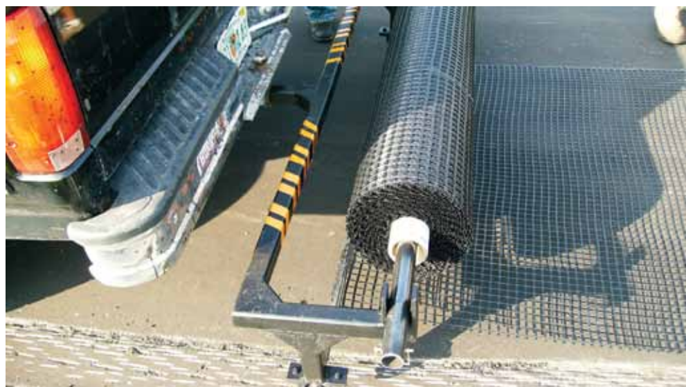
IMAGE J: GlasGrid rolls can be installed manually for smaller pavement areas.
